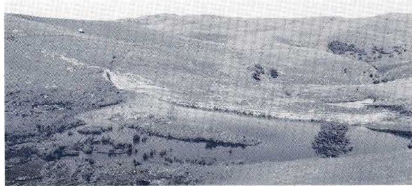
The finished pond. Downstream is the site of the next development to go ahead soon, subsidised by DU. Photo: Ken Cook.
