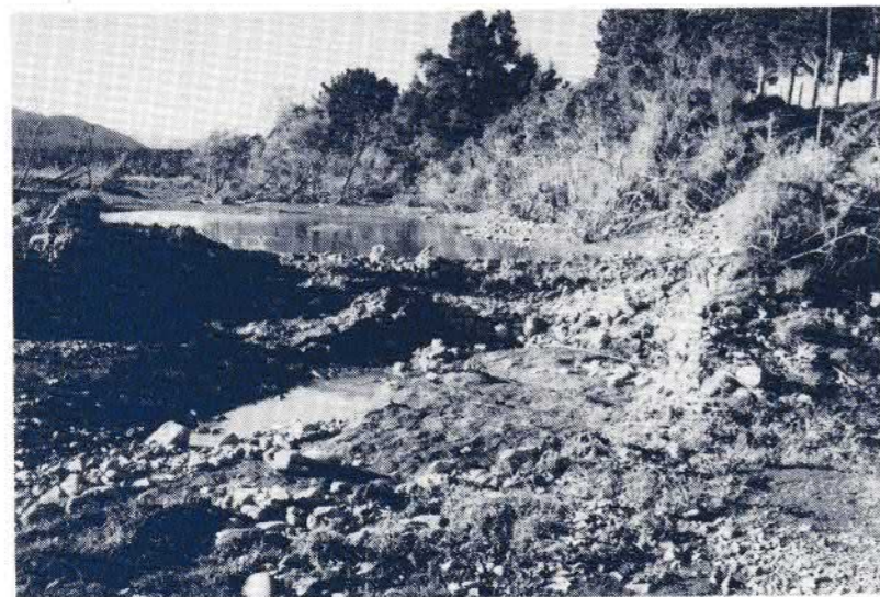
The partially repaired breach (early 1997). Photo: Alan Wilks.
