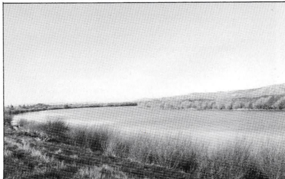
The stopbank on the Ruamahunga River prior to digging.
