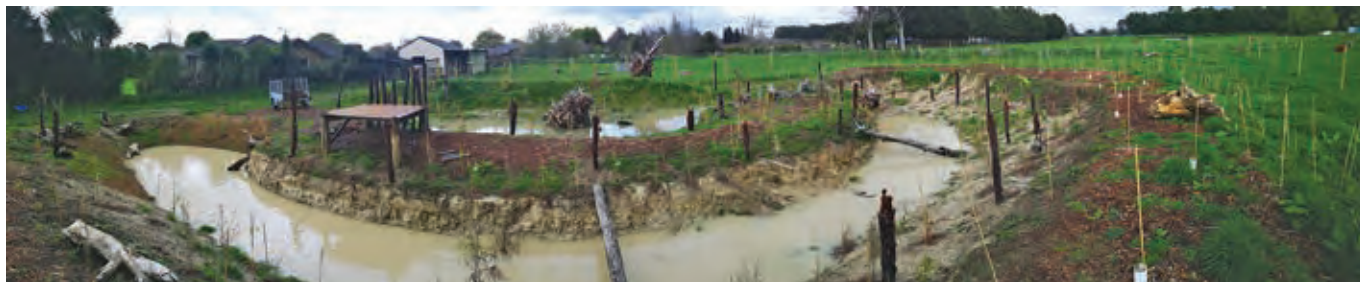
Progress in mid-September, with an observation/contemplation platform in place.
