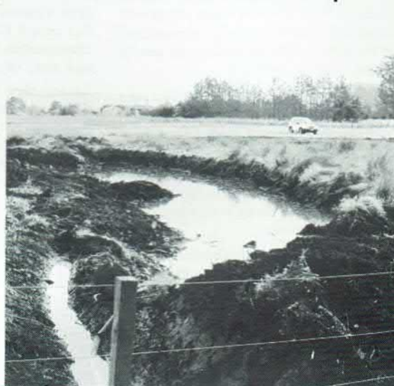
The underground pipe is found. Photo: Ross Cottle.
