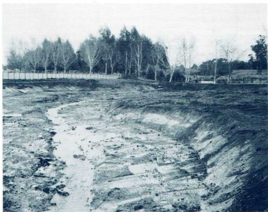
Excavation of wetland extensions. Photo: B. Butts.
