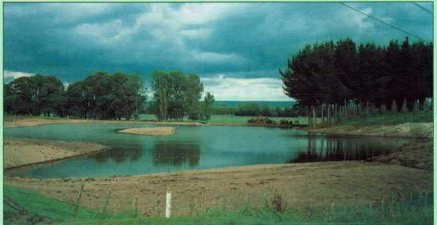
At Reporoa - a big earthmoving job costing $25,000, with planting and fencing but right beside Highway 5 promoting public awareness.
