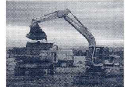
First blow of the new drain. Photo: Dennis Handyside
