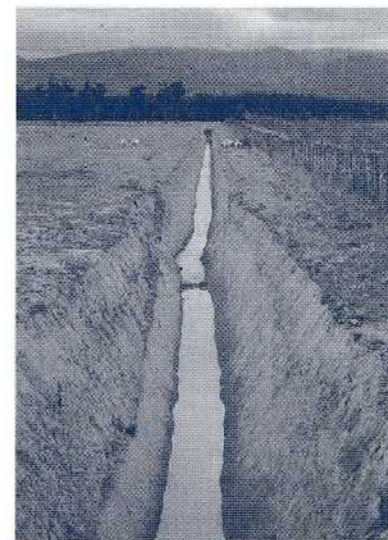
The new 400m drain carrying water to Home Lagoon. Photo: Dennis Handyside
