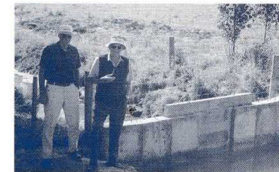
The new concrete weir diverting water to Home Lagoon. Photo: Dennis Handyside
