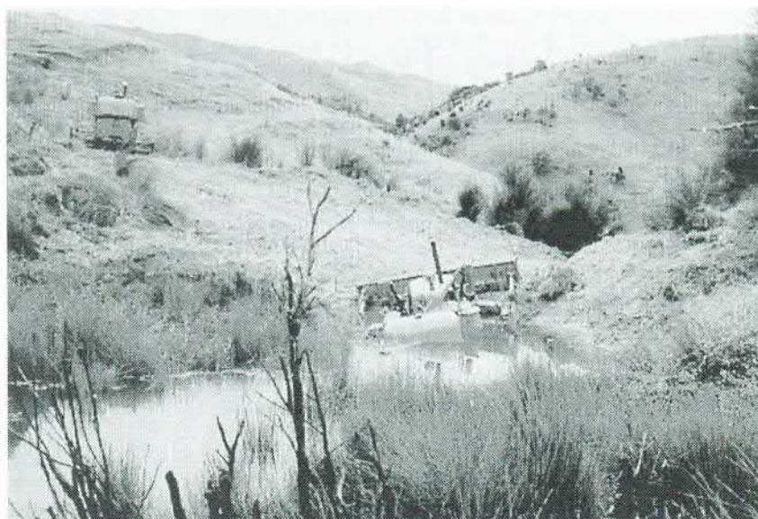
The ultimate wetland control structure. Can anyone identify this photograph?
