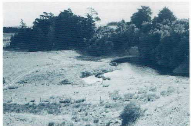
The MacKereth Wetlands at Tokomaru required the restoration of two dams lined by native bush. This is a particularly attractive development and because of the extreme water flows the spillway was sprayed with concrete for safety. The area is fully fenced and further development is planned higher up the gully.
